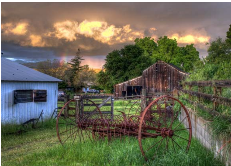
The restored West Barn (left) and the East Barn (right) before restoration.
