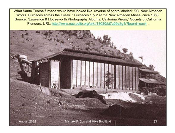
The furnace plant at the Santa Teresa mine might have looked something like this. The furnace is to the right, under the split-roof building, and cannot be seen. To the left are the tall brick condenser stacks, each an empty plastered chamber in which mercury vapor condenses, falls to the floor, and runs out to a collection trough. To the far left are the expansion chambers to reduce potential mercury mist and fume losses before exhausting the gasses to a hillside chimney.
